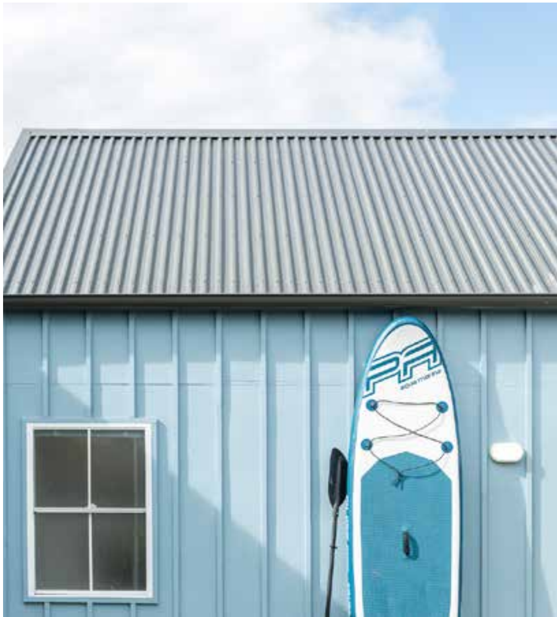
Double-hung aluminium window 1200h x 865w with colonial bars
