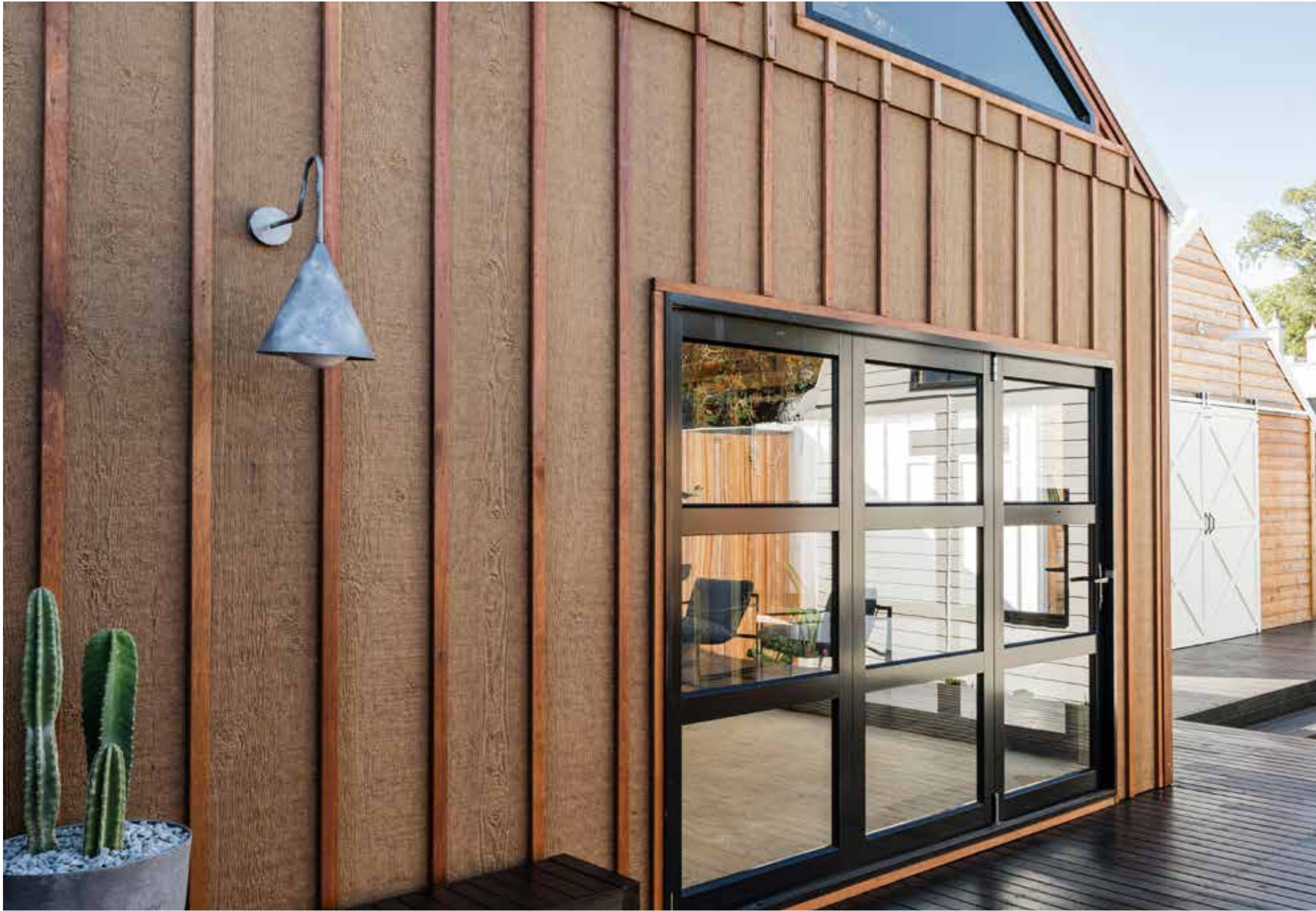
Image Left Near barn in eco-hardwood board and batten cladding Far barn in cedar weatherboard
